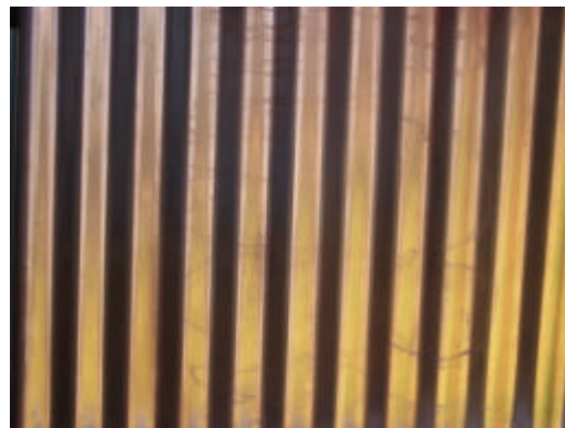
Appearance of copper roofing sheet affected by water staining (left) and after cleaning with nitric acid and Brasso (right).
