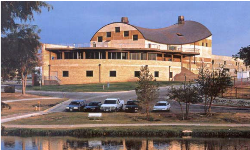
Mid-Continent Office Tower, Tulsa, Oklahoma, USA. Architect: Dewberry Design Group, Inc. Horizontal seam, 0.35 mm copper panels on a steel tube support structure.
