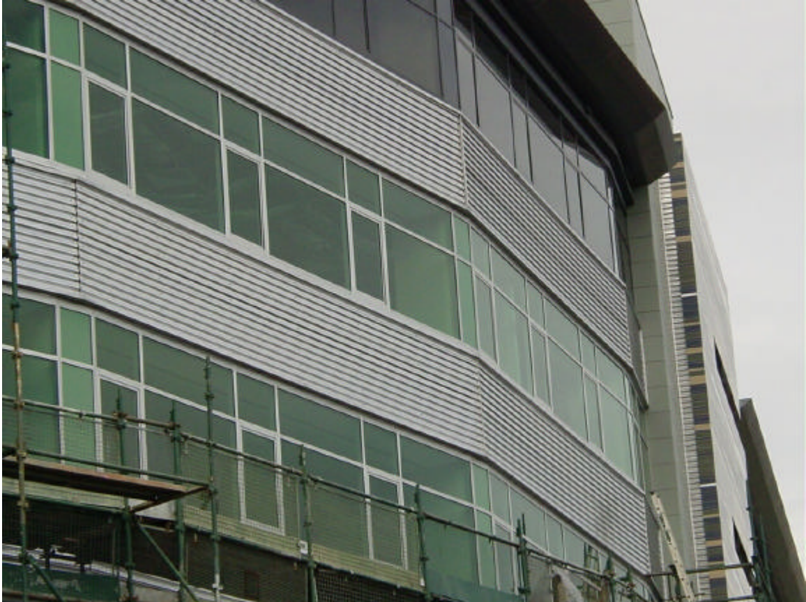
The Portal Building Development, Fortitude Valley, Brisbane. Grade 445M2 with a 2DR finish, roll formed to 'Longspan' profile.
